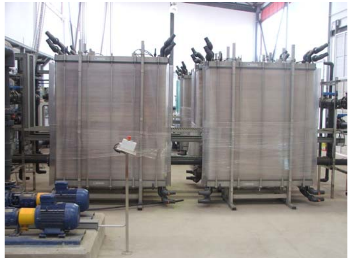
Reverse Electro dialysis stacks at Puerto del Rosario
