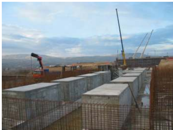
Reverse osmosis foundation
